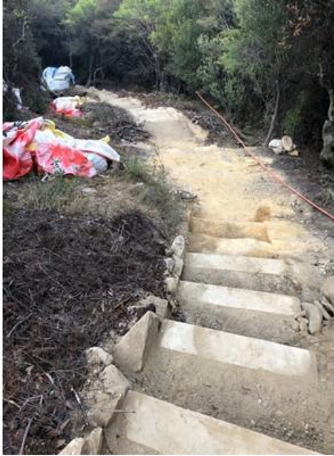
Track maintenance in near the Cascades
